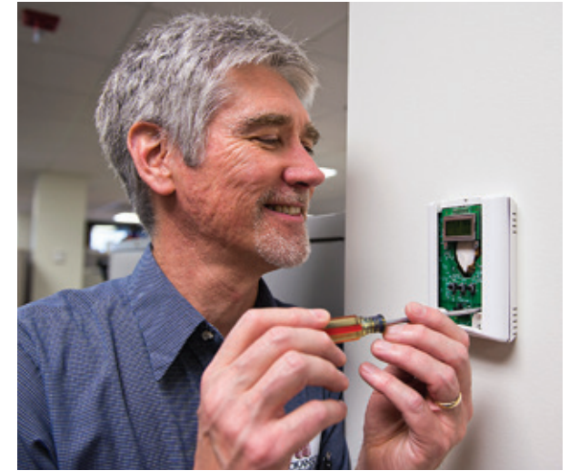
Mark McCarty of Hokanson Companies, Inc., adjusts a CO 2 detector at Old National's 123 Main Street office building in Evansville, Ind. The detectors were installed as part of a series of enhancements that greatly reduced total energy usage at the facility.
