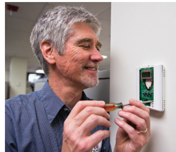
Mark McCarty of Hokanson Companies, Inc., adjusts a CO 2 detector at Old National's 123 Main Street office building in Evansville, Ind. The detectors were installed as part of a series of enhancements that greatly reduced total energy usage at the facility.
